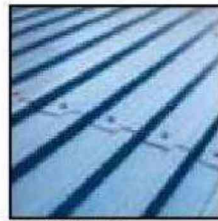
Standing Seam Metal Roof
